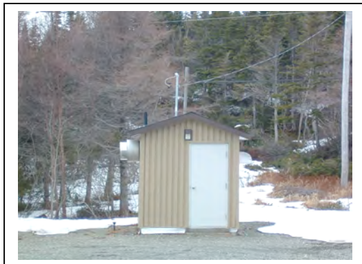
New booster station
