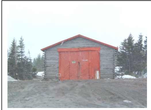
Building at incinerator/landfill site used as a kennel
