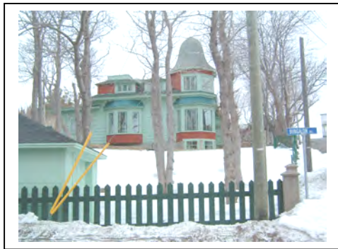
The Cabot Loop is home to many significant heritage sites and properties
